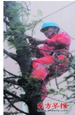
Electric Power Co. Action: repairing the wires
